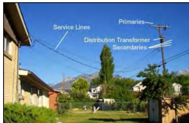
Figure 23: Household Service Line Drop from Distribution Line
