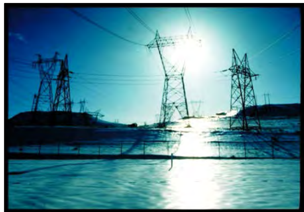
Figure 13: High Voltage Transmission Towers
