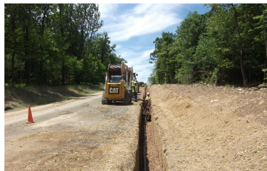
Image 5: Twin Ridges Wind Farm, Somerset, PA – underground lead line.
